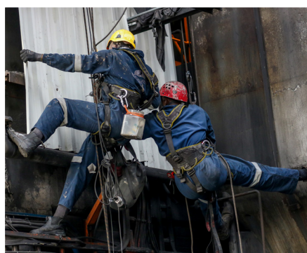
INGRAIN GERMISTON ASBESTOS REMOVAL
