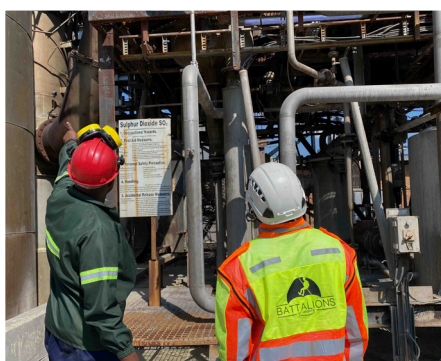
TONGAAT KLIPRIVER SO2 PLANT REFURBISHMENT
