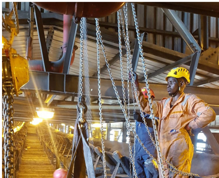
MEDUPI POWER STATION PIPE RIGGING
