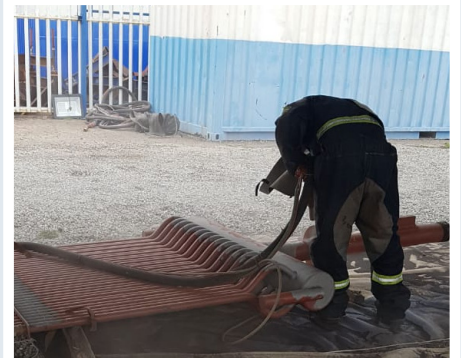
MATLA POWER STATION SANDBLASTING
